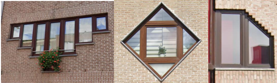
Figure 25 Zoom in first floor stepped windows of Rue de Lombartzyde 44 © Google
