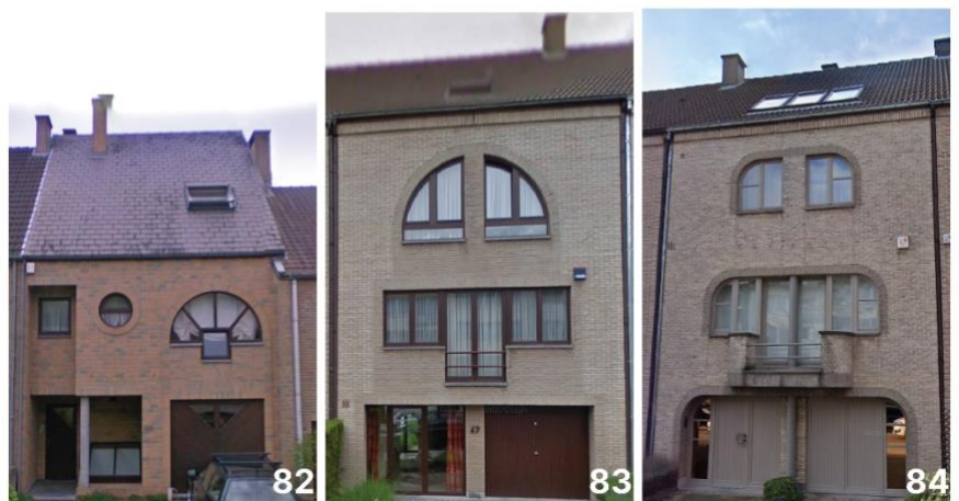
Figure 13 Selection of facades featuring particular openings © Google.
