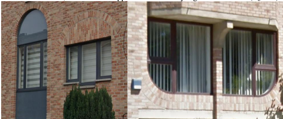
Figure 28 Zoom in curved arrangement and opening in Rue Omer Lepreux 94 © Google.
