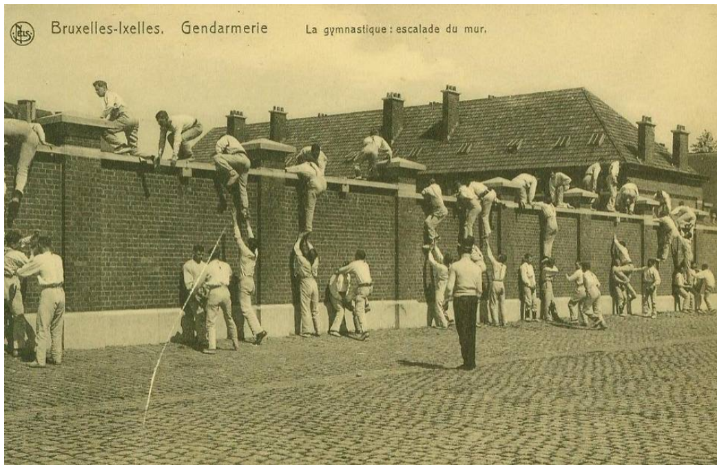
Figure 2 - Enclosure wall ©Bertrand Terlinden
