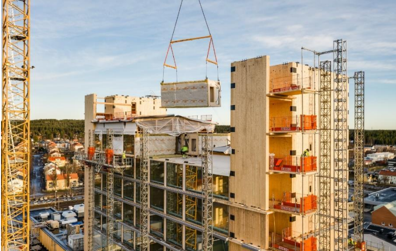
Figure 29: CLT structure of the building
