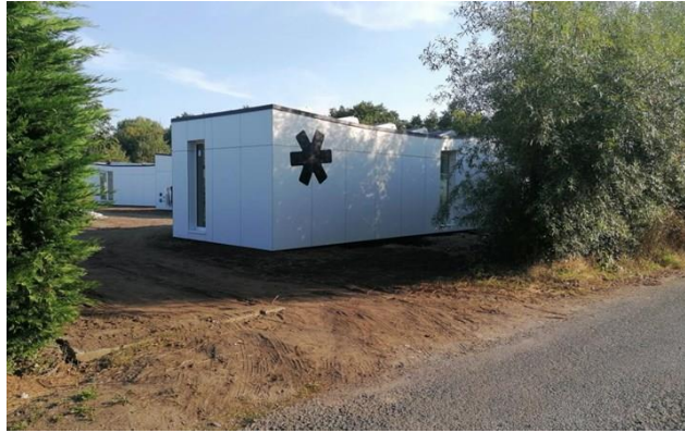
Figure 6: Transitional housing project by A2D
