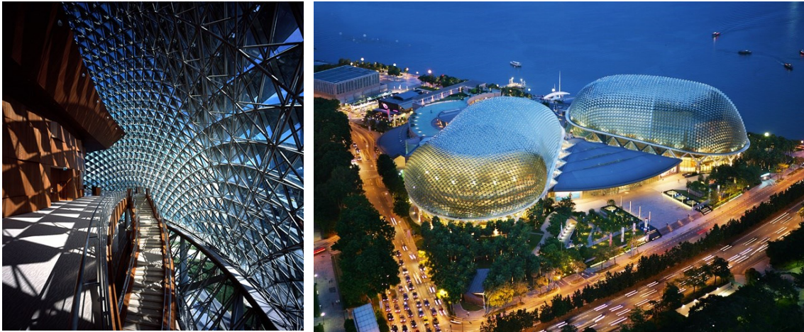
Figure B - 6: Left: Inside view on the shell structure and glazed envelope with shading. Right: View on the two rounded envelopes by night (DP Architects Pte Ltd. 2020).
