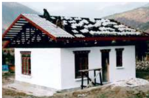
Figure 20: Microconcrete (MCR) roof tiles produced on site, cheaper than CGI sheets; here also with a ventilated roof. Architect Chris Butters. (Butters, 2015)
