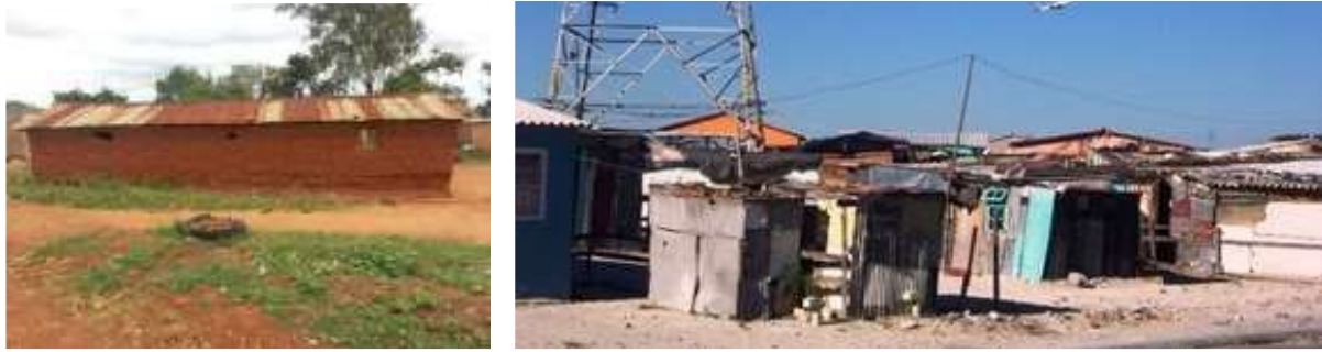
Figure 19: Examples of CGI sheeting in hot climates. Left: Typical rural house construction in Tanzania. Right: Typical slum housing with CGI roofing, Capetown, South Africa. (Butters, 2015)
