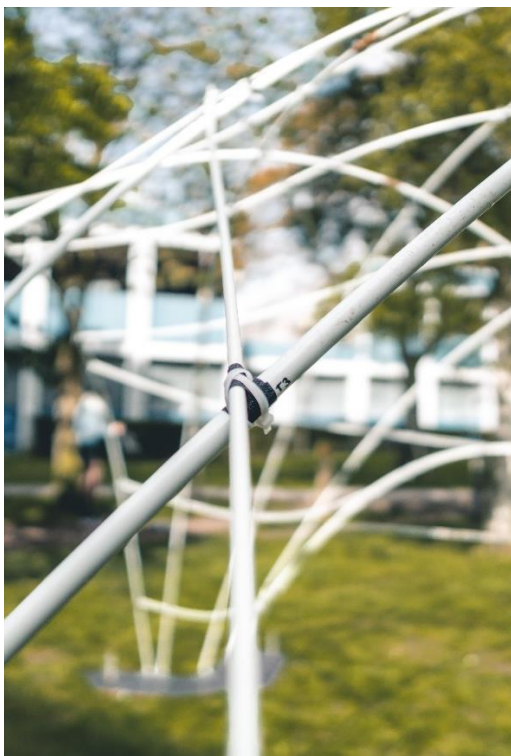
Figure 82 : Photo of the nodes realized, (a) Crossing node, (b) Boundary node
