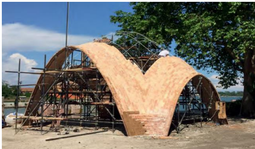
Figure 60 : Construction of the drone port in Venice, 2016 16
