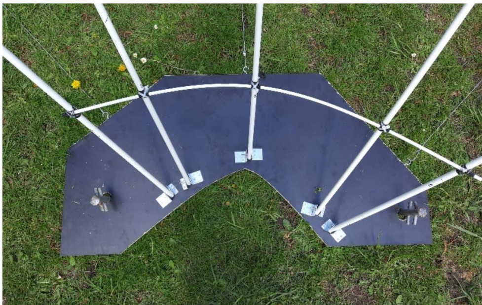
Figure 89 : Final anchoring of the gridshell
